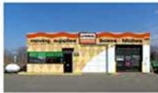
Facility re-imaging on schedule
